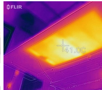
Figure 4. IR image of infrared heater.
