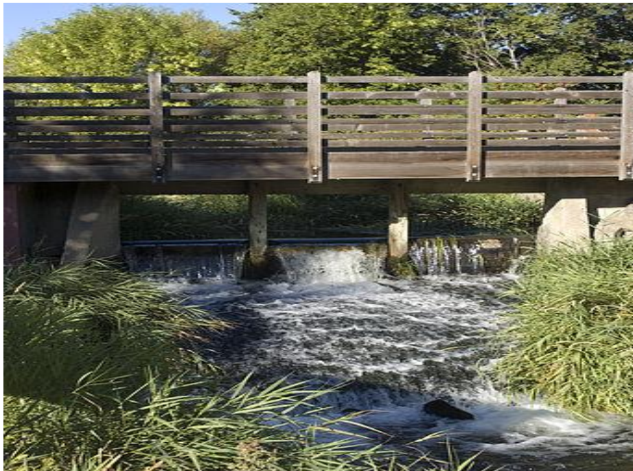
Figure 1-1 A broad-crested weir at the Thorp grist mill in Thorp, Washington, USA.
