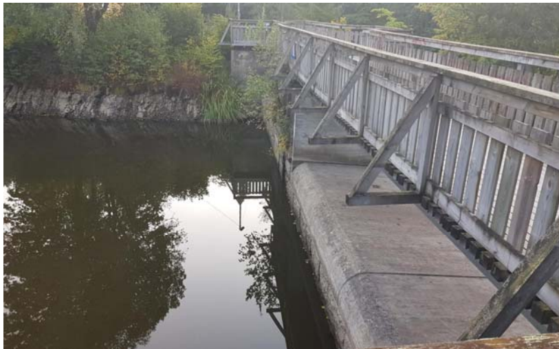
Figure 1: Example of a broad crested weir with roundly shaped edges
