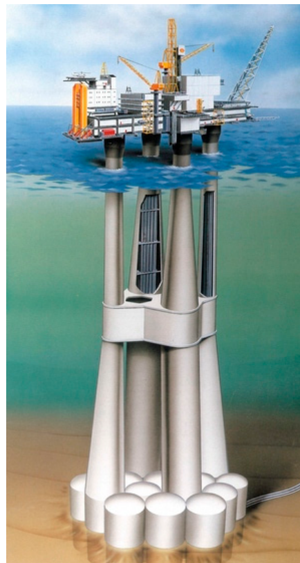
Figure 2. An example of Condeep oil storage platform: Troll A [3].
