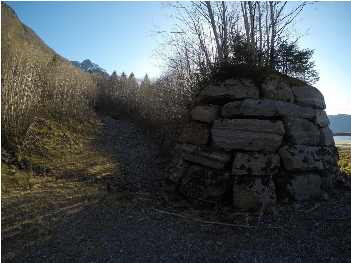
Figure 13: Deflection wall along E39, Flåskjer, Ørsta
