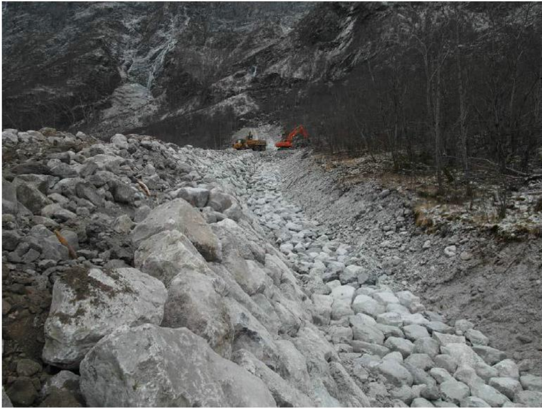
Figure 21: Erosion protection in Hallinggrovi, Norway (Høydal & Kronholm, 2013, p. 48)
