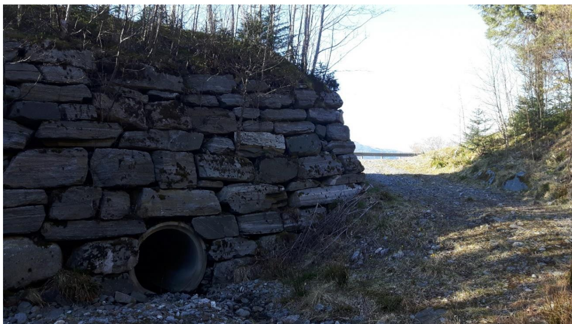
Figure 20: Culvert through a deflection wall along E39, Flåskjer, Ørsta
