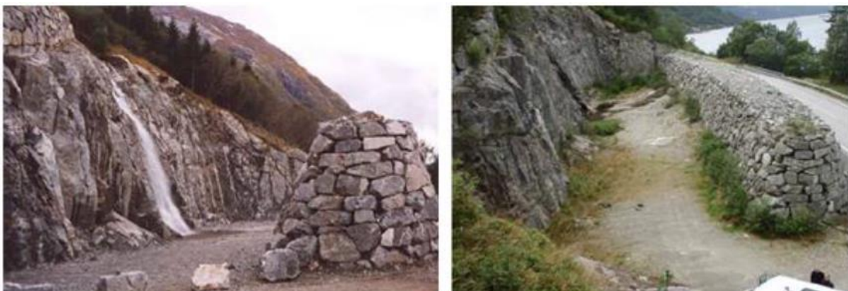
Figure 22: Terminal wall in Norway (Norem, 2011, p. 90)
