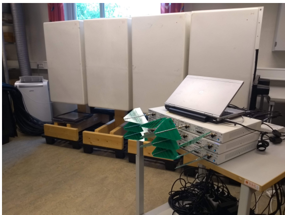
Figure 4.1: Test setup, Base station antennas in background and user terminals in foreground.
