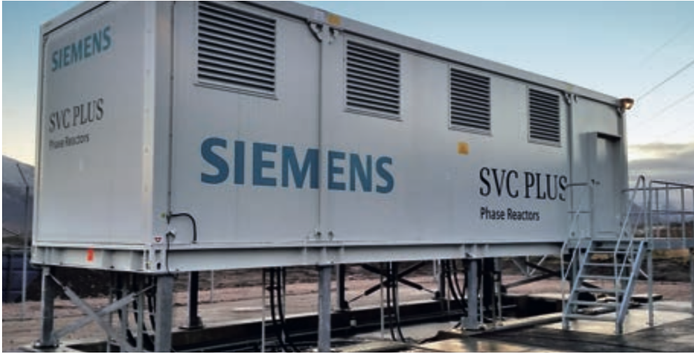
Figure 2.4: STATCOM installed at Sortland [11]
