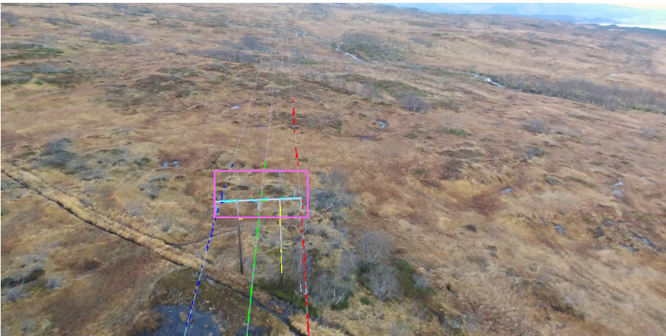
Figure 4.3: Power mast detector result
