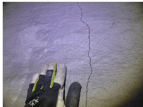
(f) Not corrosion classified as Red corrosion, rebar by networks 3,4,5, 8 and 9.
