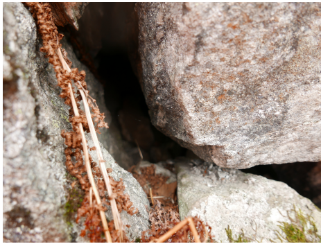
(a) Not corrosion classified as Red corrosion, steel construction by all networks 2-9.
