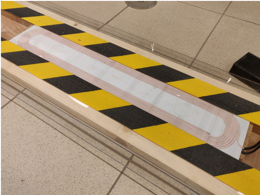
Figure 2.7: A closer look at one of the induction coils.
