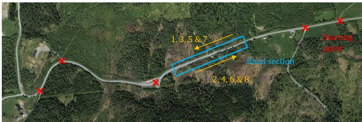
Figure 26: Picture showing the road section
