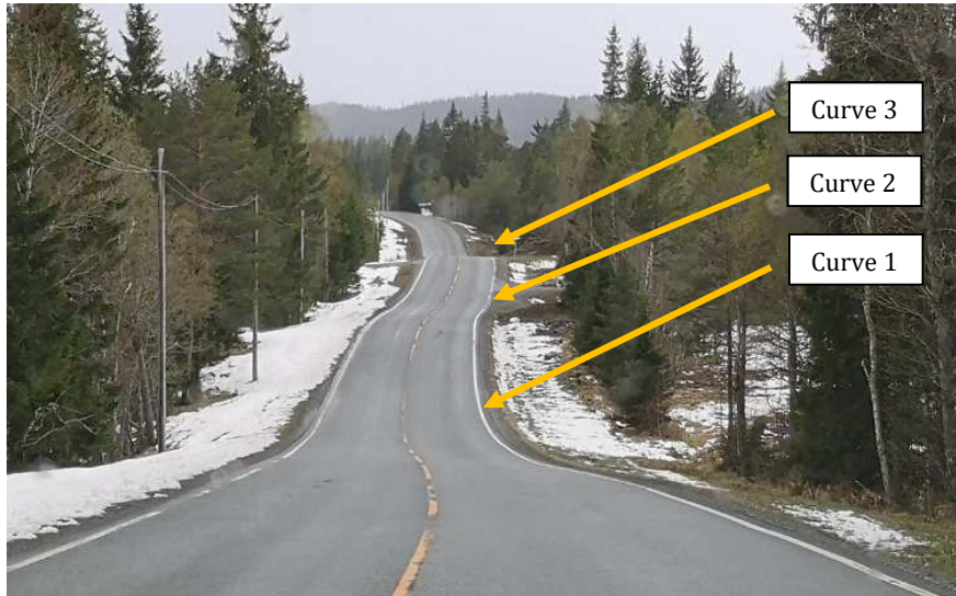
Figure 27: The road section showing the alignment (south-west direction). The picture shows curve 1 and curve 2, with curve 3 behind the second crest curve.
