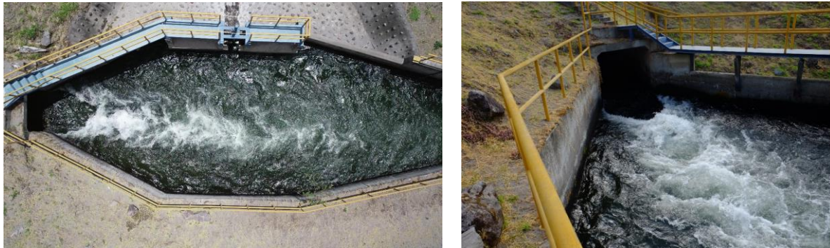
Figure 3-6 Aerial view of desander (Left) and Inlet of the desander (Right)
