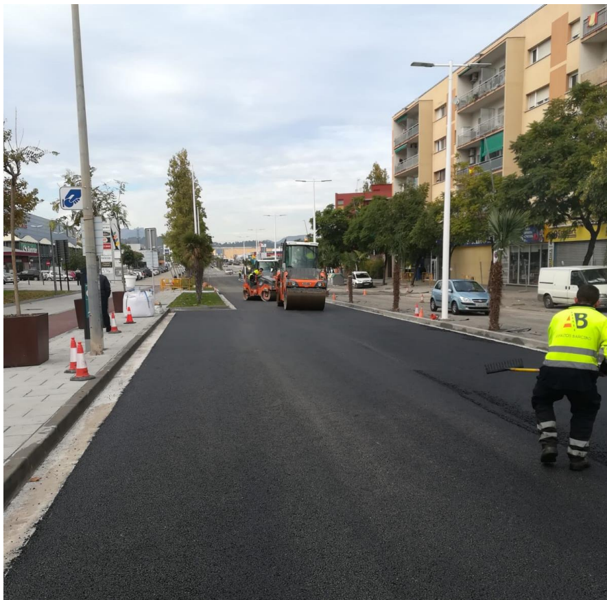
Figure 4.27: Carrying out asphaltting tasks on the road (Civil Stone)
