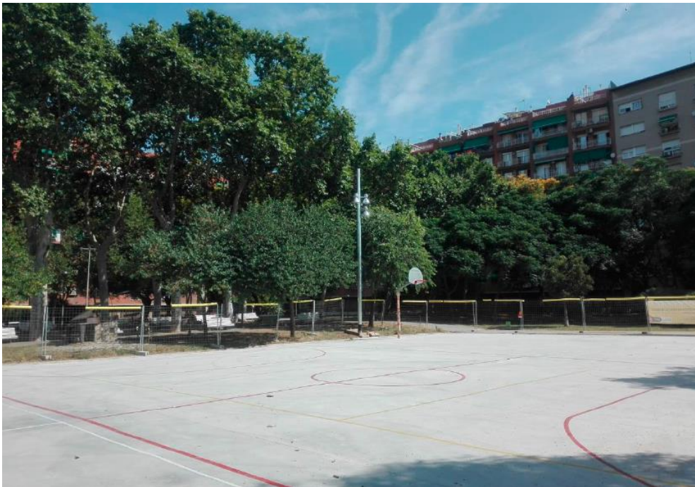
Figure 4.16: Final result of the performance in the basketball court (Civil Stone)
