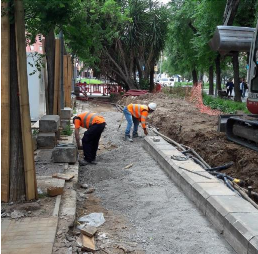
Figure 4.14: Workers performing tasks in the parterre (Civil Stone)
