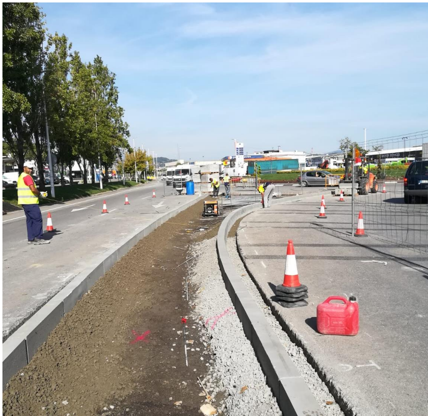
Figure 4.26: Workers performing tasks in the new median strip (Civil Stone)
