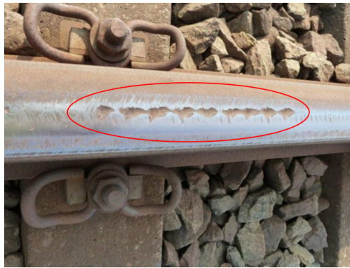
Figure 2.6: Spalling surface flaw (Steenbergen, 2016)
