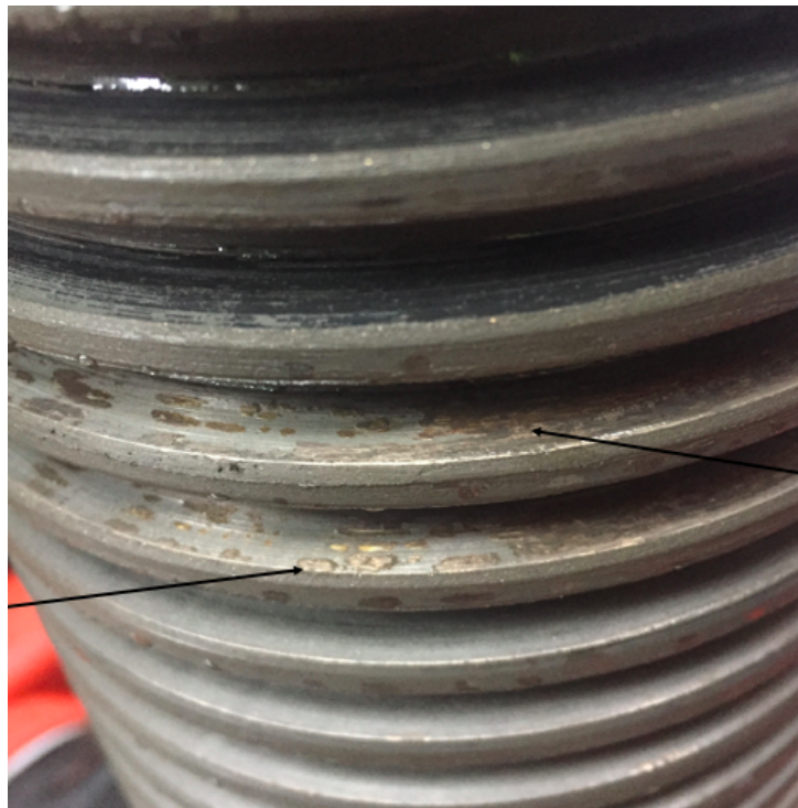
Figure 3.17: Photograph of the full-scale xylan coated SDSS power screw after operation for 43 days at Fosen harbour. Arrows are given to show examples of areas of degraded coating.
