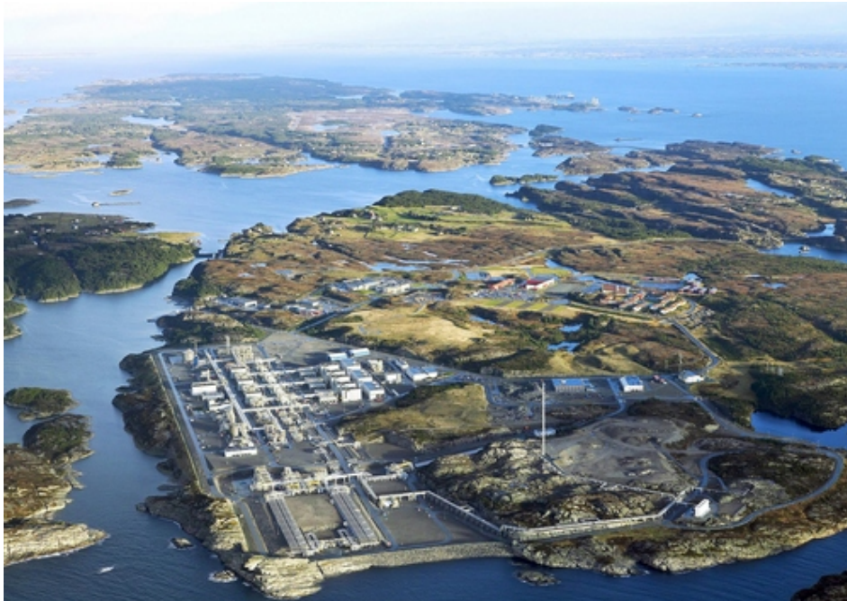
Figure 3.1: Picture of the gas processing plant at Kollsnes[74].
