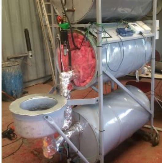
Figure 21: The second setup after pipe insulation and removing the pistons
