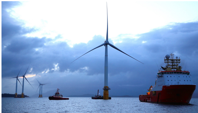
Figure 1.8: Transportation of Hywind turbines [13]
