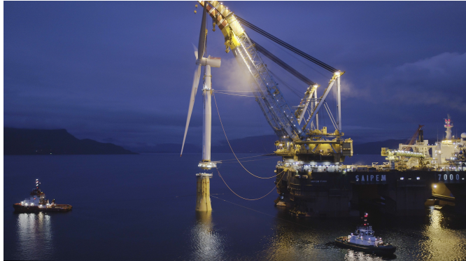
Figure 1.10: Lift operation Hywind Scotland [16]
