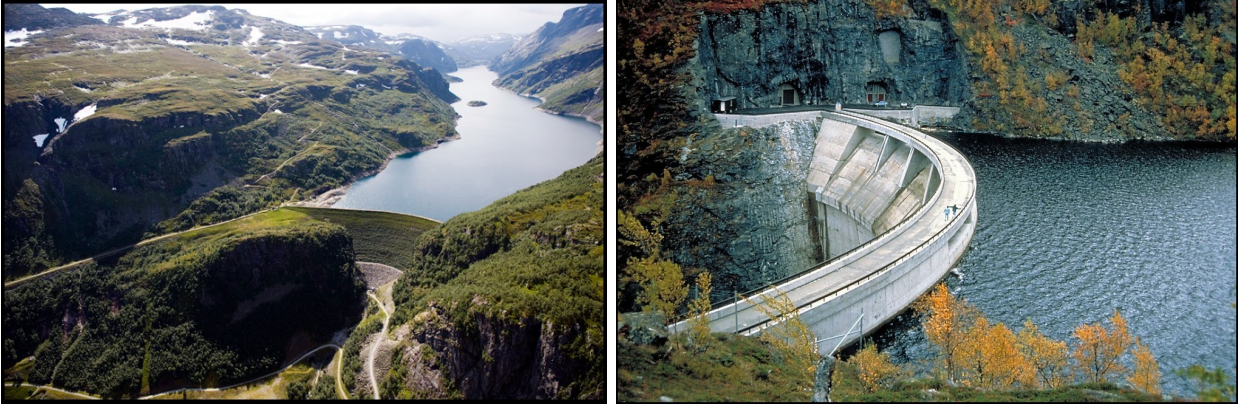
(a) Barrier dam at Aurland I Power Plant [13]
