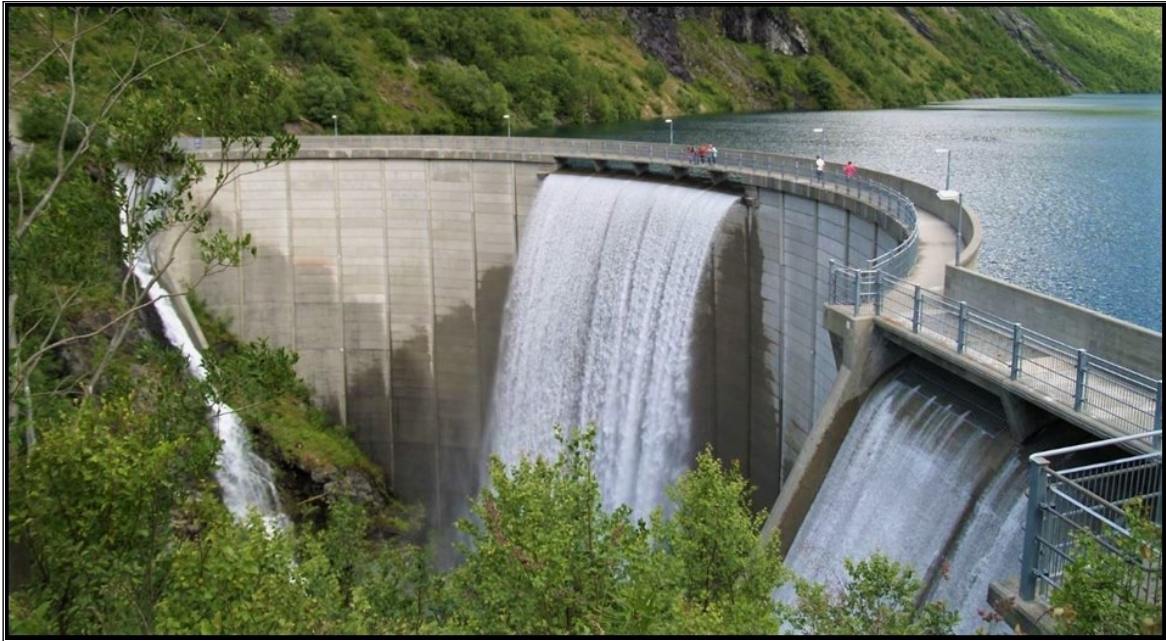
Figure 3: The Zakarias Dam, Second highest magazine dam of Europe. Taken from [12]
