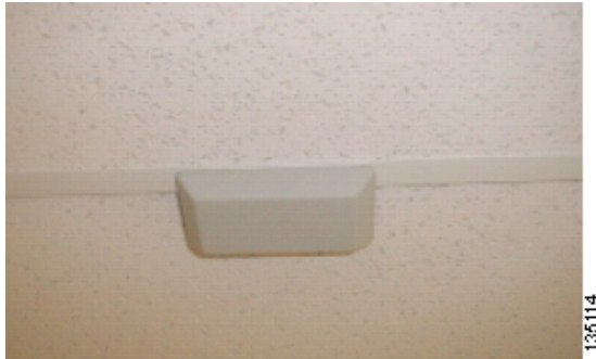
Figure 5-6 Patch Antenna Mounted on a Suspended Ceiling
