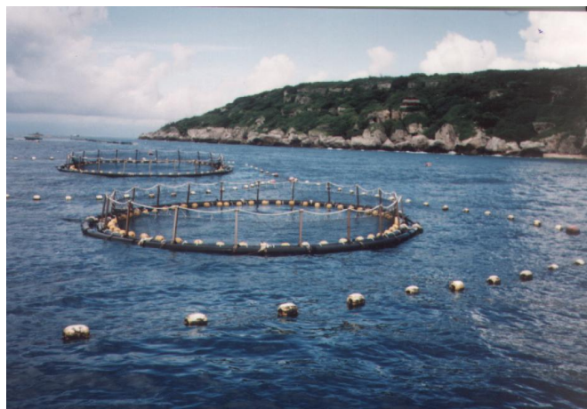
Figure 2-3: A flexible sea cage [5]
