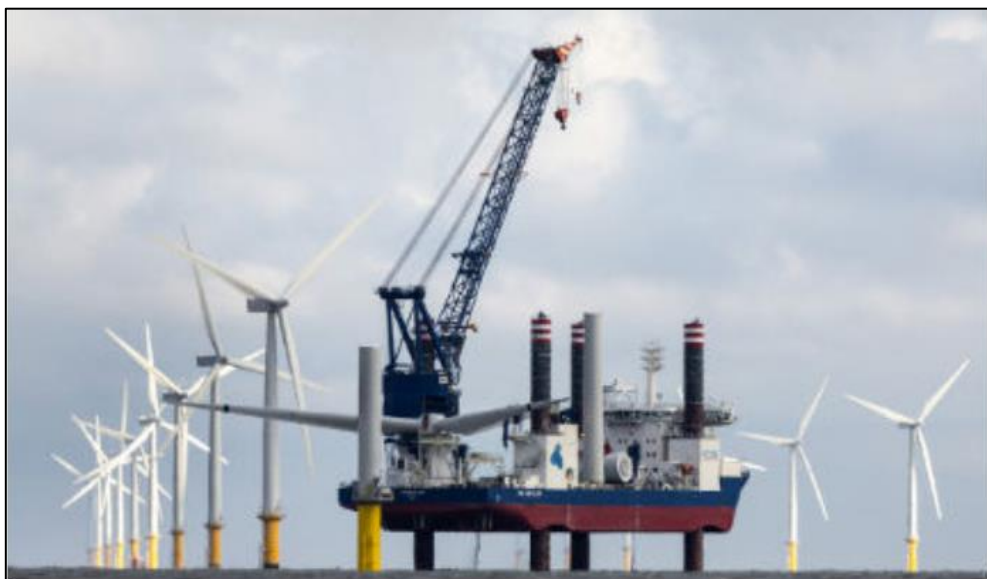
Figure 2:1 Jack up barge installing the wind turbines in a wind farm (8)
