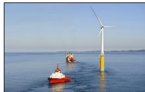
Figure 1.1: Left: Installation of OWT on spar fundament. Right: Towing of the complete assembly to mooring site.
