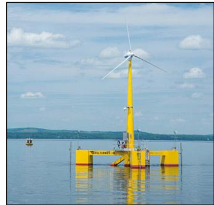
Figure 2.1: Three-column semisubmersible test platform.
