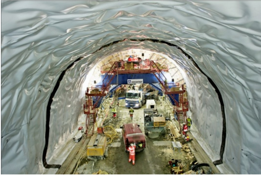
Figure 2.2: Installation of sheet membrane in the Ulvin Tunnel (Ausland and Jonsson, 2014).
