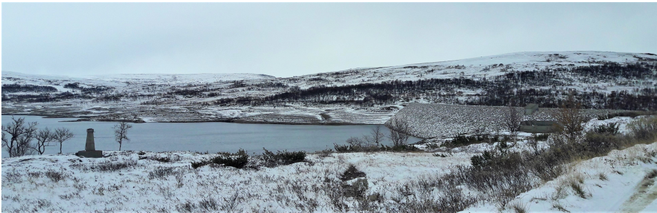
Figure 6.2: Falningsjøen embankment dam seen from the reservoir on the left side.
