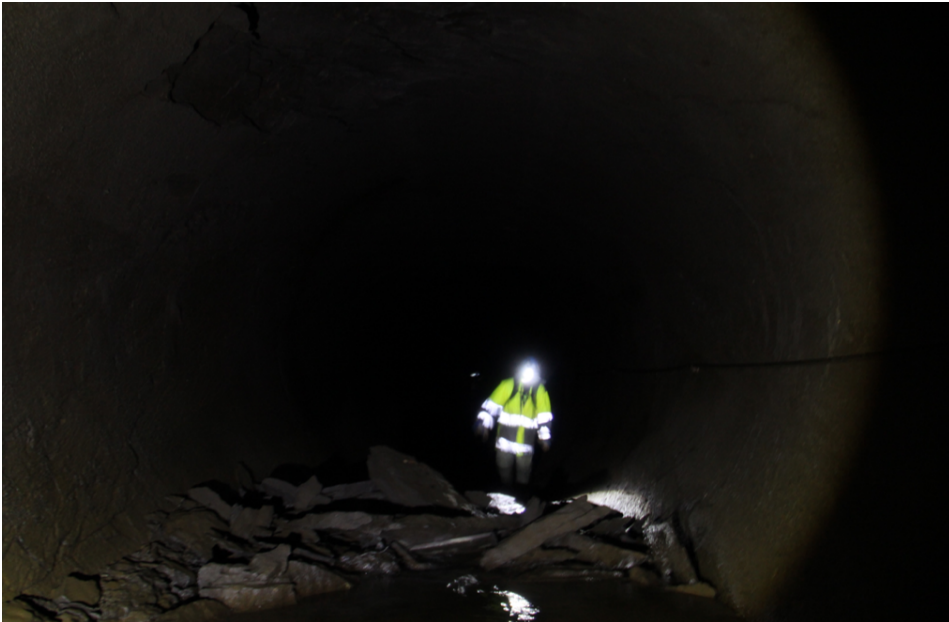
Figure 10.4: Rock fall due to stress induced failure in the crown 6230 m downstream of the CSS.
