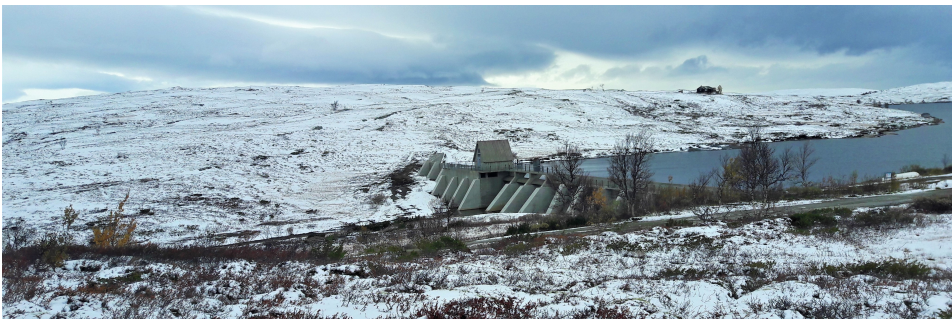
Figure 6.3: Sverjesjøen buttress dam seen from the right side of the reservoir.
