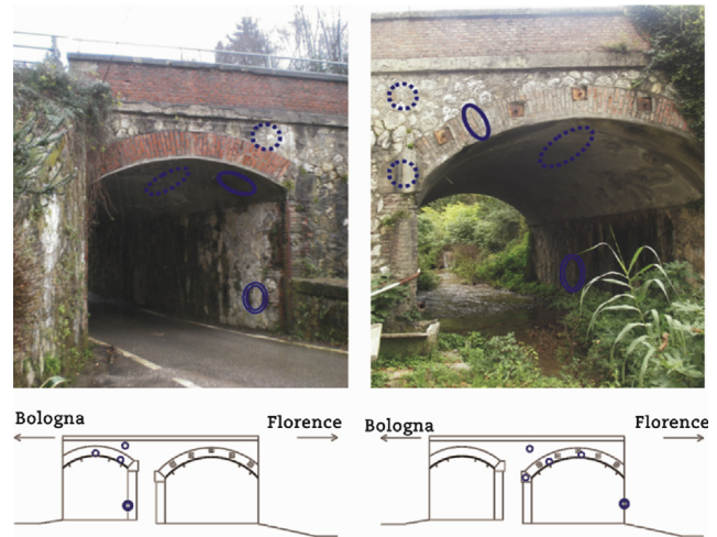
Fig. 3 – Position of the executed tests: single flat jack (single solid line), double flat jack (double solid line), core drilling and boroscopy (dashed line).
