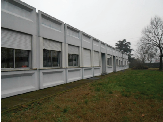
Fig. 1. Southwest façade of the child care centre.
