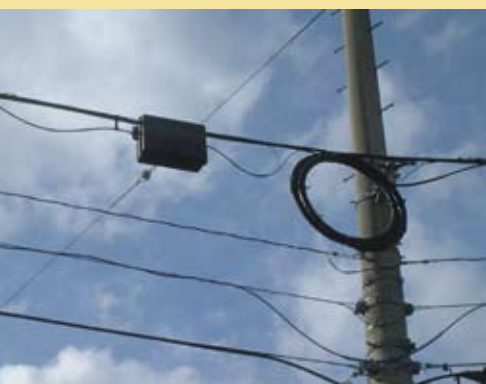
Distribution box for fiber lashed to existing aerial cable; this method is quick and inexpensive.
