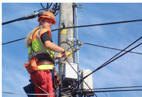
Example – Aerial Feeder Cable Installation
