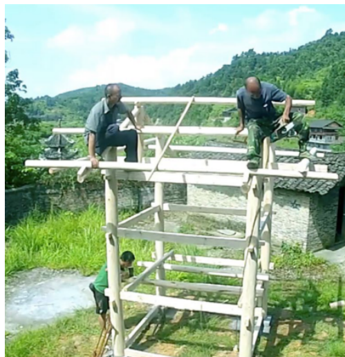
Figure III- 3, local construction works (W. Wang et al., 2016)
