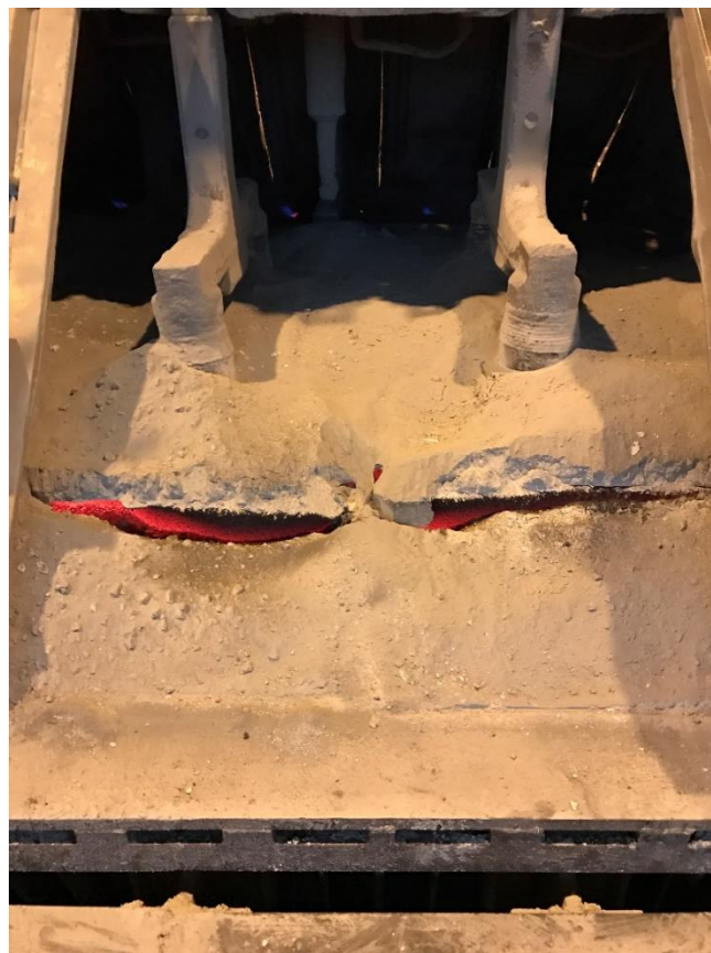
Figure 3.1: Access area to the pot interior when two pot covers are removed.
