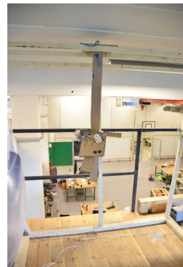
Figure 13: Second ceiling console.
