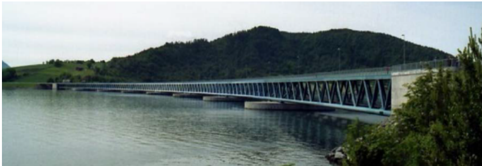
Figure 1.2: Bergsøysundet Bridge (Villoria, 2015)
