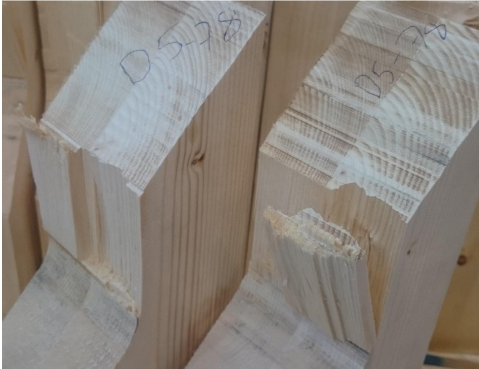
Figure 45-Partially Independent fracture of a 2 lamella specimen, notice the change in fracture over the adhesive zone.
