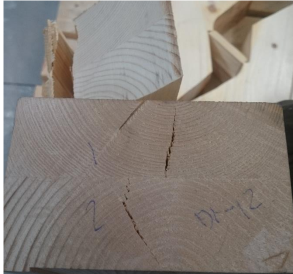
Figure 2 - radial cracks in both lamellas in a radial Longitudinal test specimen D1-12.
