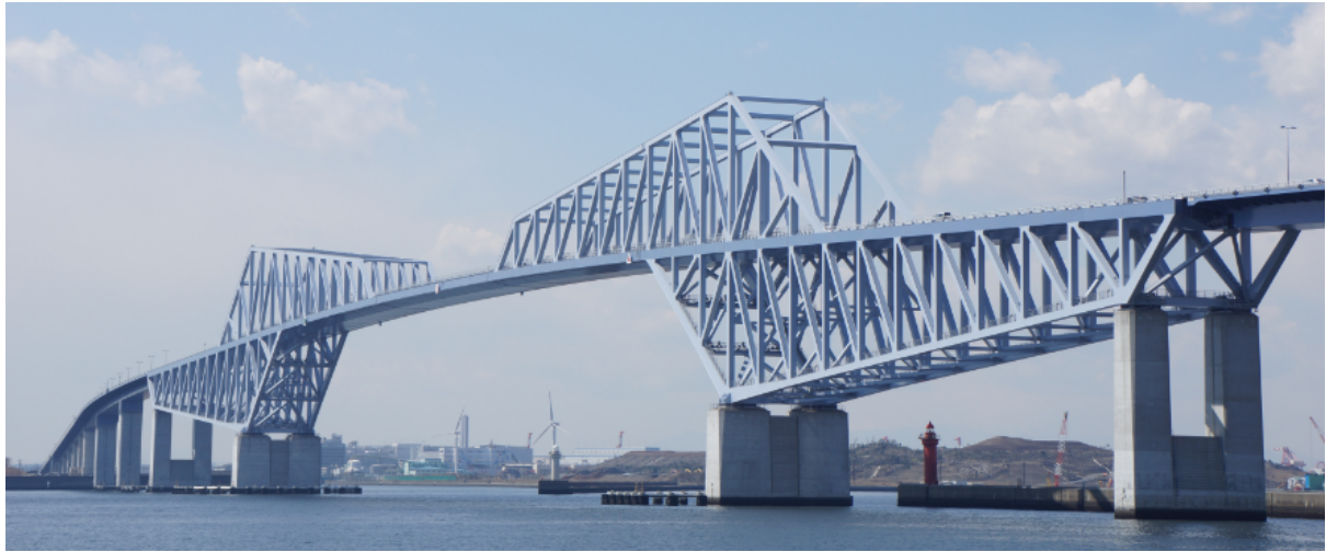
Figure 4.15: Tokyo Gate Bridge.
