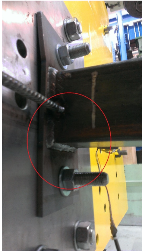
Figure 9.18: The bottom of the RHS profile of specimen A
