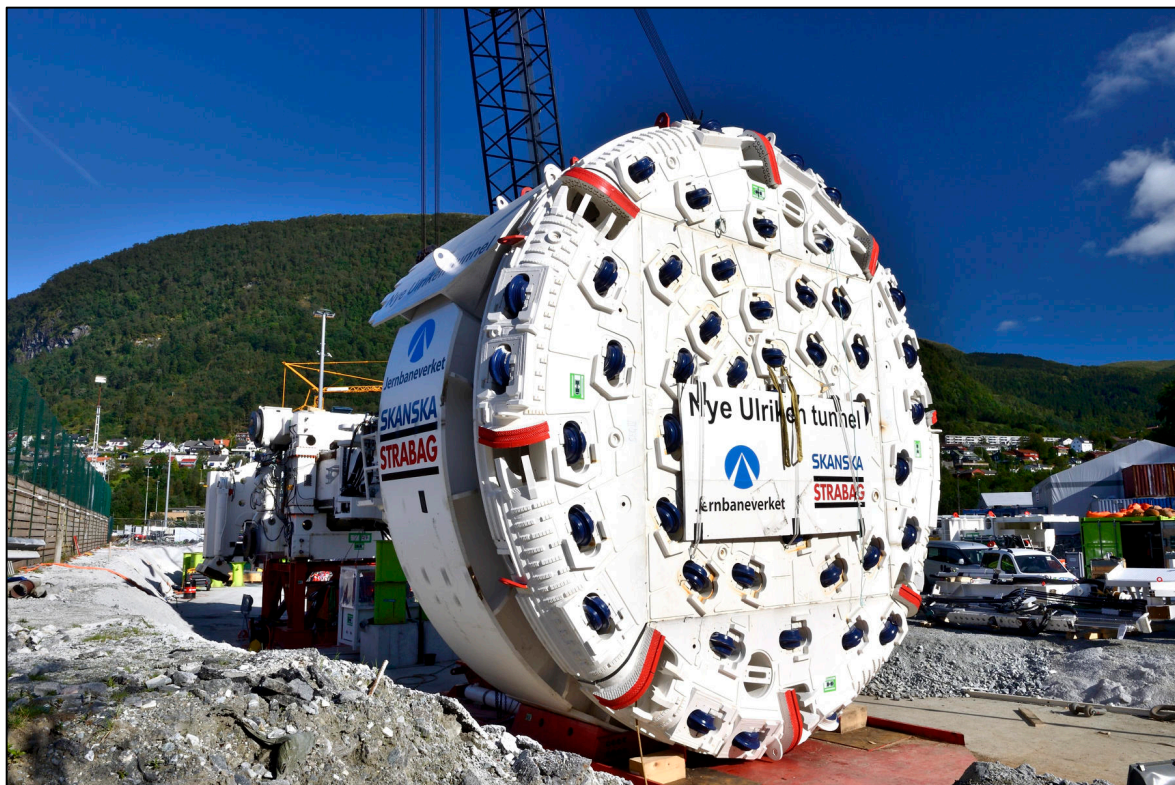
Figure 2.6 The TBM for the New Ulriken Tunnel (Photo: Øystein Grue)
