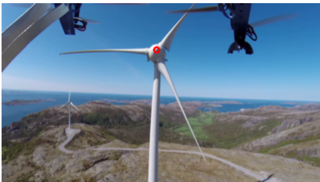
Figure 6.10: The red circle shows the estimated hub center position calculated from the average of the intersection points from figure 6.8.
