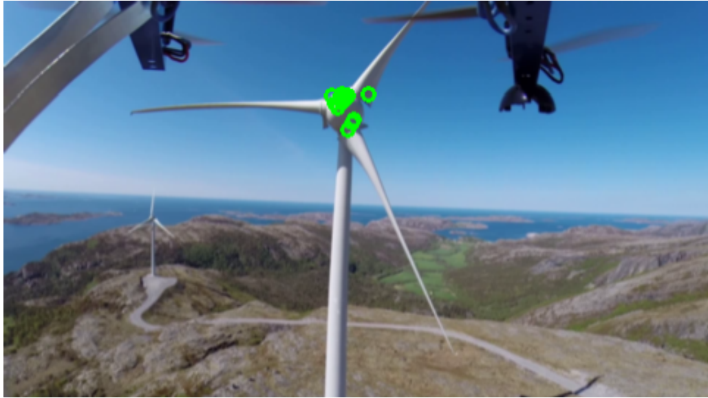
Figure 6.8: The green circles show the points where the blade lines intersect each other.
