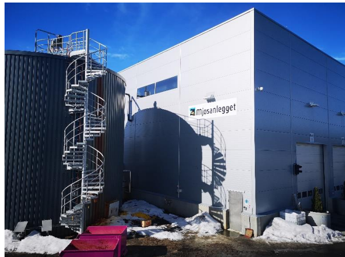
Figure 1: Mjøsanlegget's main operative building and buffer tank.
