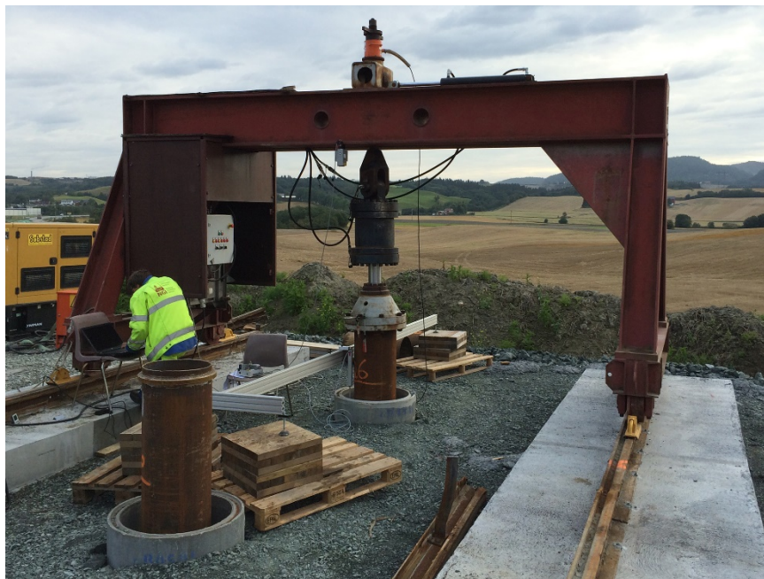
Figure 31. Pile test reaction frame. Image modified from [65].
