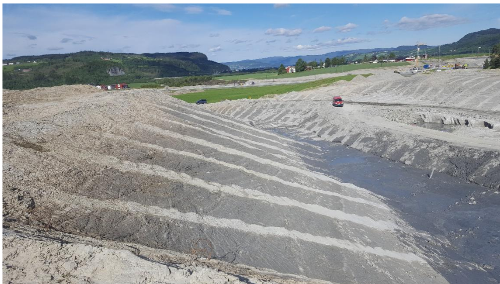
Figure 36. Lime cement column ribs constructed at Klett.
