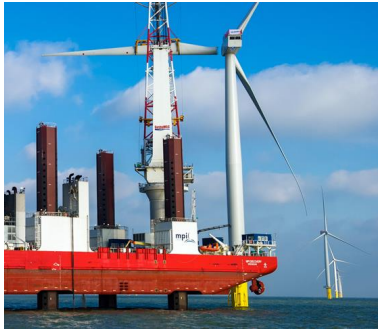
Fig. 2. Horizontal lifting of blade [16]
