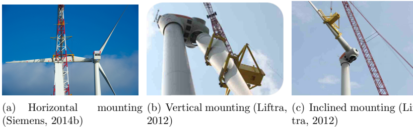
Figure 1: Single blade installation of offshore wind turbine blades with various orientations
