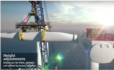
(c) Step 3: the blade root approach the hub [91]
