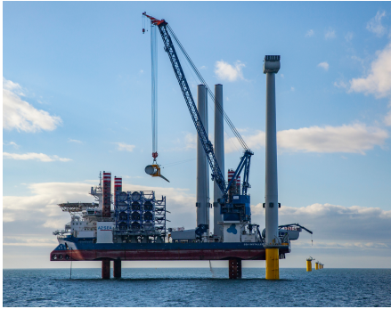
(a) Step 1: lift the blade off vessel deck [7]
