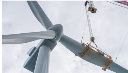
(e) Step 5: mate the blade root into the hub [80]
