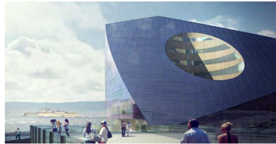
Figure 6: Powerhouse Brattørkaia in Trondheim, Norway. Upon completion, this building will utilize building integrated photovoltaics for electricity production.
