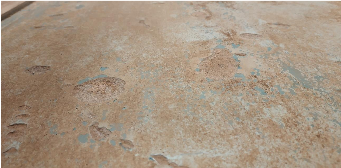
Figure 44 Detail of the concrete bed of experimental flume
