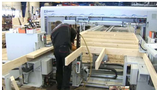
M.0101 – framework construction
