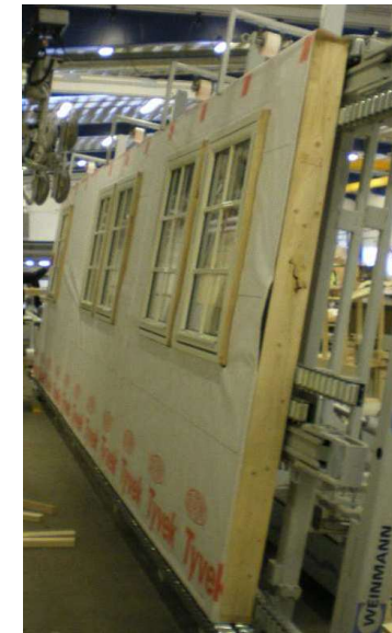
M.0103 – window installation
