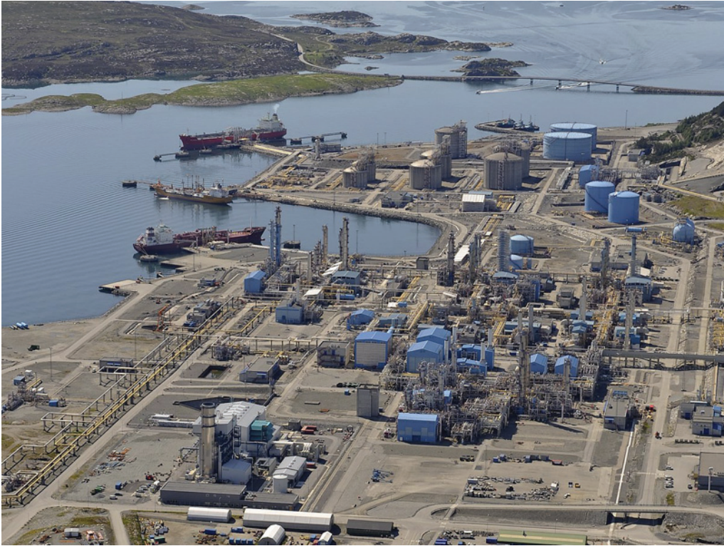
Figure 1.1: Kårstø gas processing plant. Photo: Statoil.
