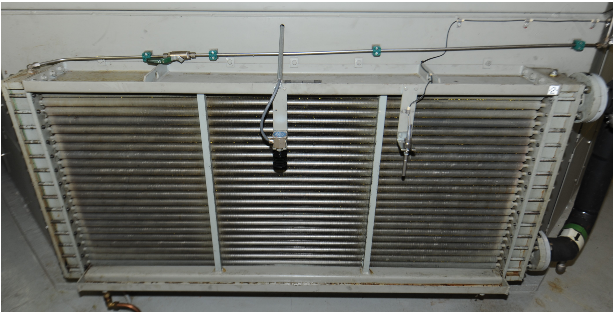
Figure 2.5: Generator air cooler at Brattset hydropower plant, received from TrønderEnergi
