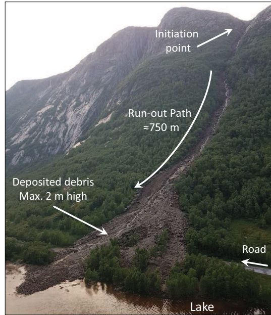
Figure 1. Example of a debris-flow in the coastal areas of Norway [Hunnedalen, Norway - occurred on 2 June 2016]. (Courtesy: Multiconsult and NPRA).
