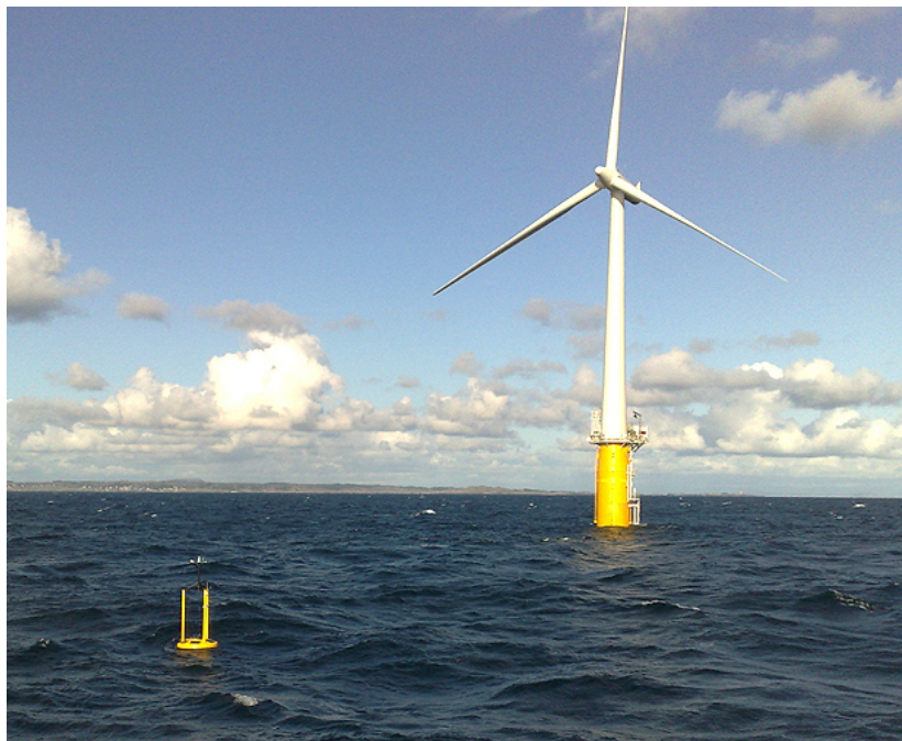
Figure 1. Hywind in Åmøy Fjord, the first full scale Offshore Floating Windmill
