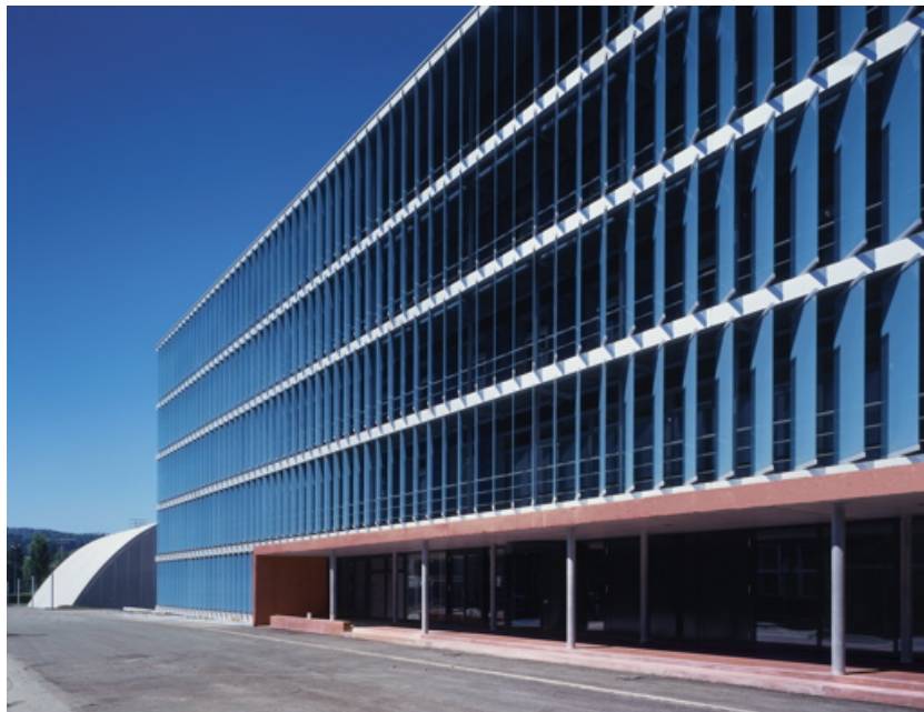
Figure 1.4: The vision is to design a control system that is applicable in all existing and new office buildings. Source: OptiControl.
