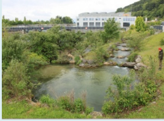
Photos: Nature-like bypass channel for fish, and rock-cascade fish pass (both photos Pinja Kasvio)
