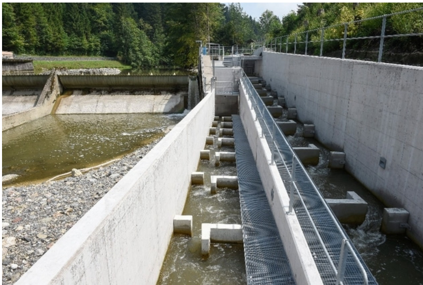
Fish pass at Hüttener Wehr (EKZ) in the river Sihl, Canton Zürich/Switzerland. Photo: André Springer.
