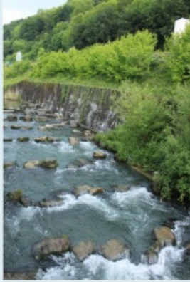
Photos: Nature-like bypass channel for fish, and rock-cascade fish pass (both photos Pinja Kasvio)
