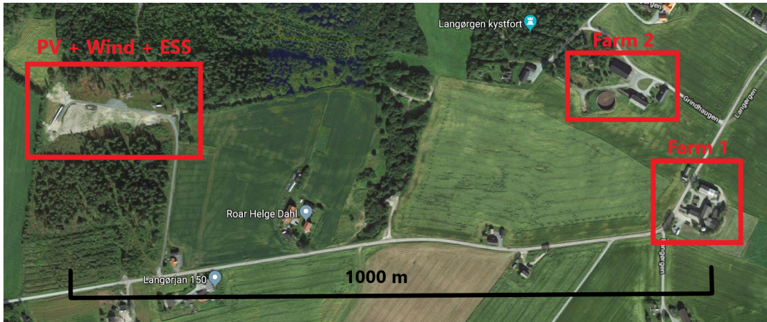
Figure 2.3.1: Overview of the sites that constitutes the microgrid. There is a 1 km long transmission line between the power producing units and the farm sites.
