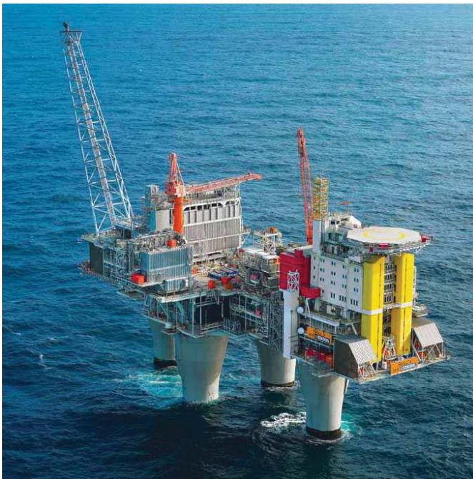
Figure 1.1: The offshore Statoil Troll A gas platform located in the North Sea. Note the large living facilities on the right, which is required due to the large number of workers on the platform. Courtesy ABB Strategic R&D for Oil, Gas and Petrochemicals.
