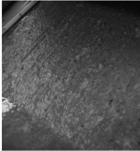
Figure 1.6 Thick filter mat on a rotating belt sieve with a mesh size of 350 \mu\text{m} at the Breivika WWTP (Rusten & Ødegaard, 2006).
